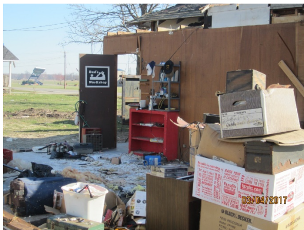
The occupant in this home was behind the brown wall when the storm hit.
